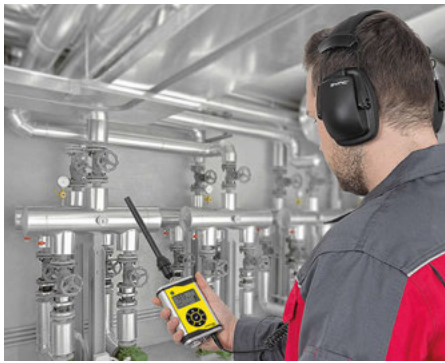
Using the directional sound probe, leaks at exposed lines can be located precisely.
